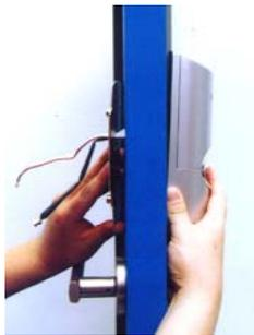
Insert the outside unit's wire (Main P.C.B connect cable and Fingerprint module connect cable) to the above hole, and insert it to the steel plate hole of the inside unit.
