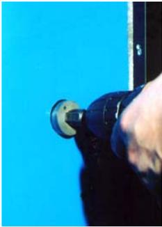
Punctuate a hole using 30~32mm hole drill. The position of the front and back holes may have some tolerance.
