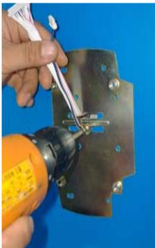
Fix the steel plate of the inside unit and the outside unit using two bolts, but do not tighten them fully. After confirming that the inside unit and outside unit are aligned, tighten them fully.
