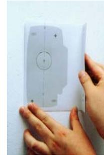
After determining whether the door is a right-hand or left-hand door, fold the template to fit the hole by an angle of 90 degrees. This product can be used regardless of whether you have a right-hand or left-hand door.
