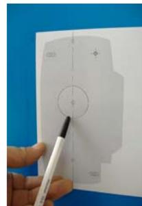
Mark the center hole position of the template and the bolt position of the latch with a pen or center punch.
