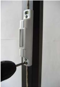
If the gap is appropriate, fix the latch onto the screw hole that had already been marked. Check if the door lock automatically locks when the door is closed.
